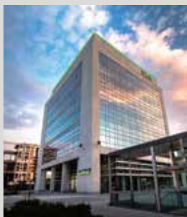
HQ Mansion of DKV, Spain
